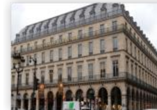
巴黎会议大厦 Paris conference building
